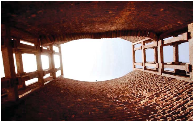
Vaulted walls for tank construction
