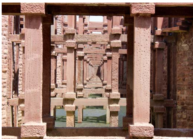
Series of storage tanks similar to 'Bawari'
