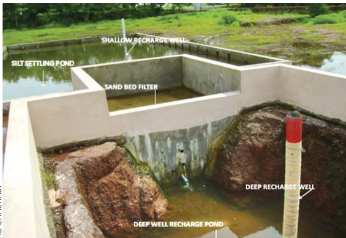
RWH structures – deep trench, sand filter and recharge well
