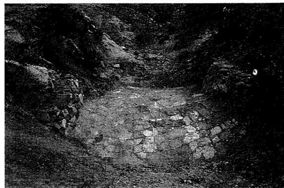
A weir constructed with effective involvement of people holds water (photo 1), while another weir lower down constructed earlier was always dry (photo 2). Note the wall protecting a large area in photo 1.
