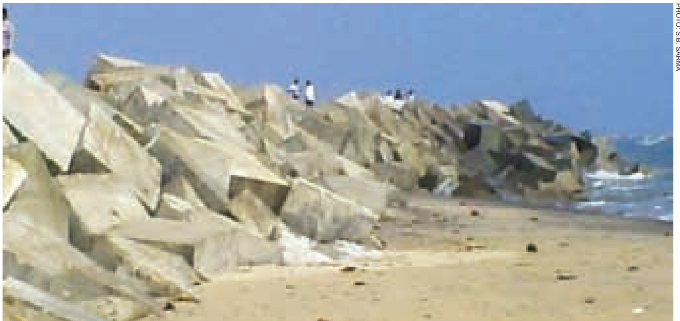
Figure 9.9.3: Attempts to save Uppada's shore using RCC blocks
