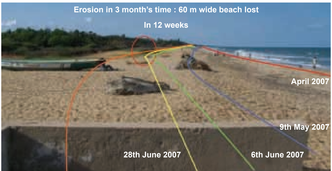
Figure 5.24: Shoreline change north of groyne field
