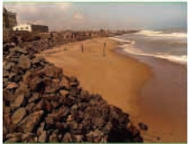
Figure 6.22: Sea wall along Rayapuram. (Source: MoES 48 ).
