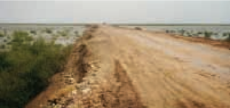
Figure 6.13: Road construction under way for proposed satellite port at Tuna 29
