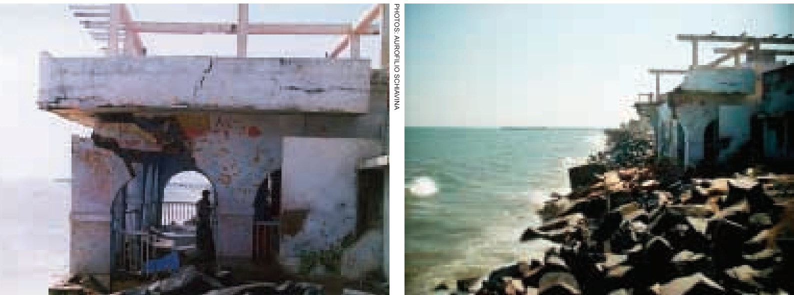
Figure 5.18: “Le Café” building collapsing into the sea due to coastal erosion
