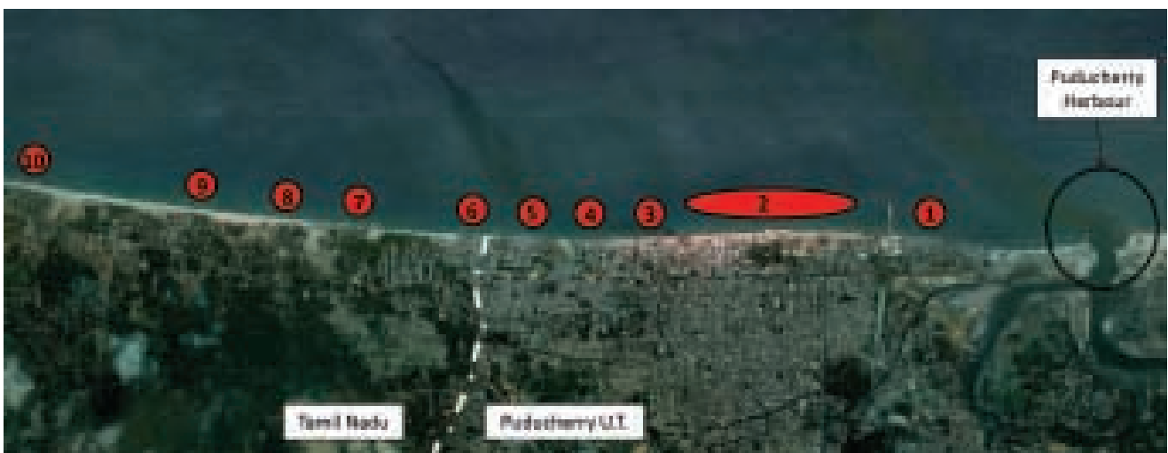
Figure 5.29: Coastal settlements affected by coastal erosion caused by harbour
