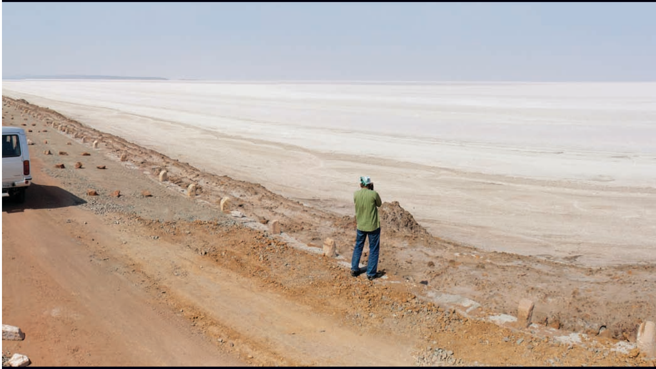
The bridge across the Great Rann of Kachchh, connecting Khadir Island to the Indian mainland
