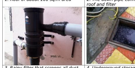
3. Rainy filter that screens all dust 4. Underground storage tank of particles more than 200 micron size 1000 lt. capacity
