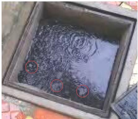
Dust particles got clustered and floating on the water surface in storage tank (immediately after a rainfall event)
