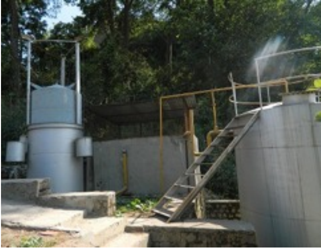
The existing plant at PD (Prep Department) was refurbished under the directions of Clover Organic Pvt. Ltd. The plant now offers water quality within CPCB norms including the Coliform count.
