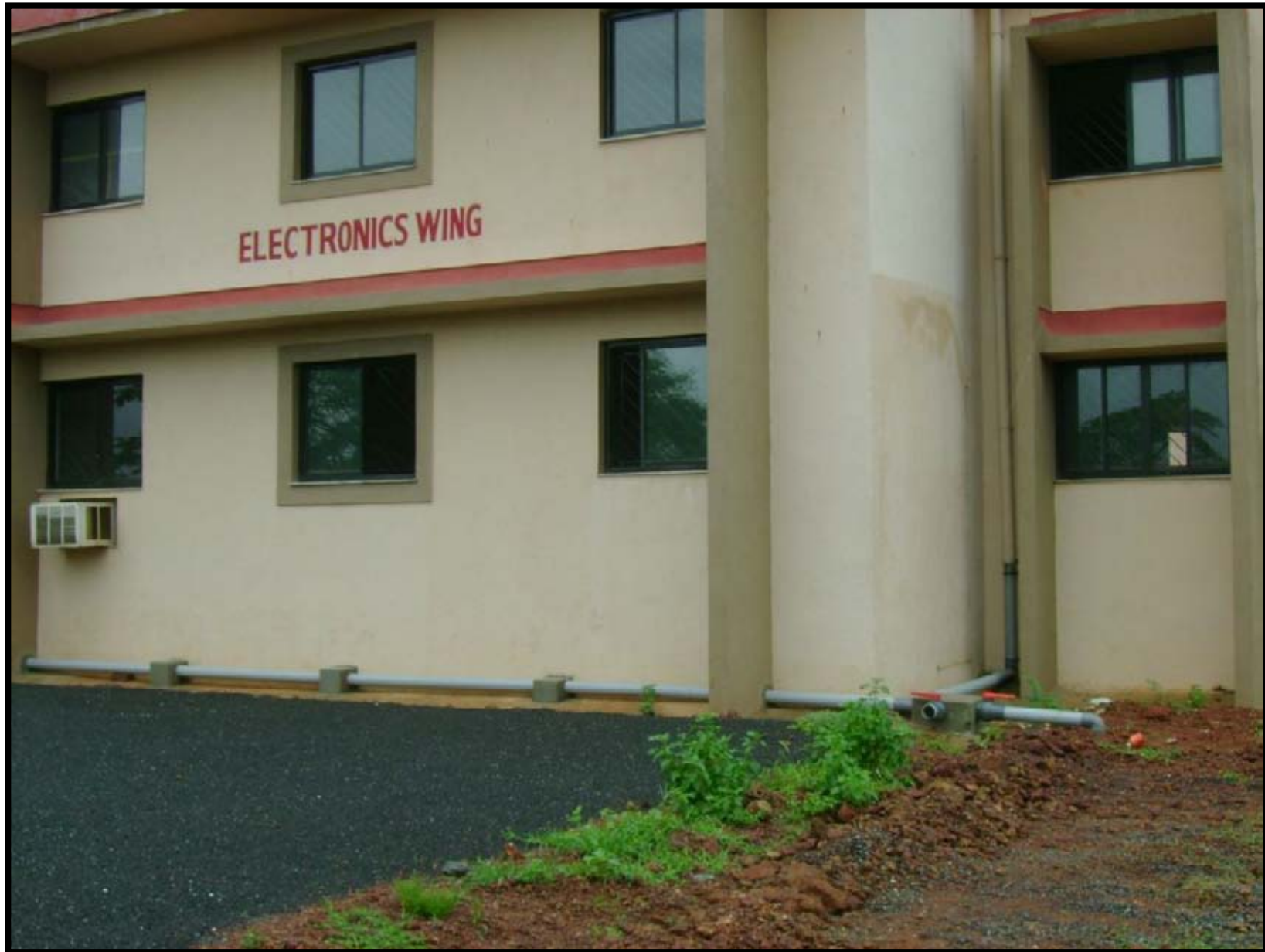
Roof water coming down through special PVC pipes
