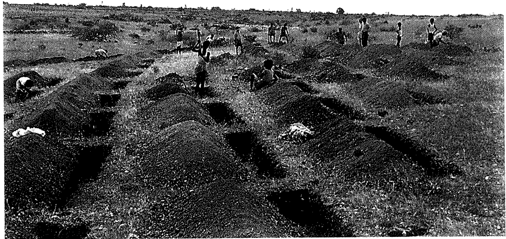
Deep Trenches on Waste Lands
