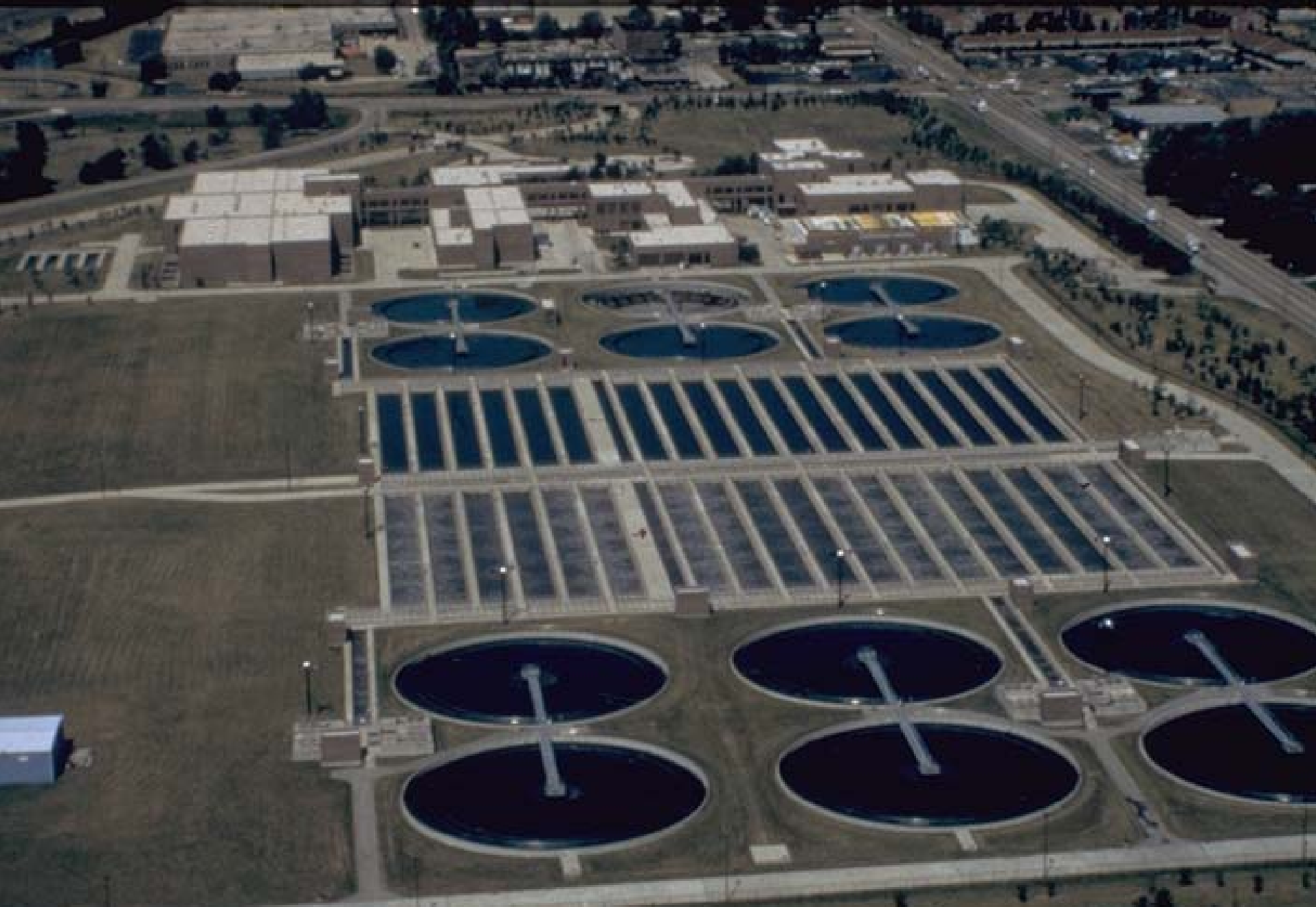
James C. Kirie Water Reclamation Plant
