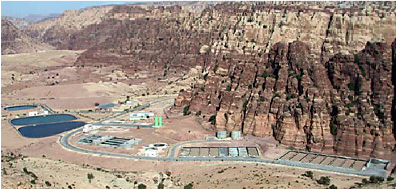
The Wadi Mousa Wastewater Treatment Plant in Jordan
