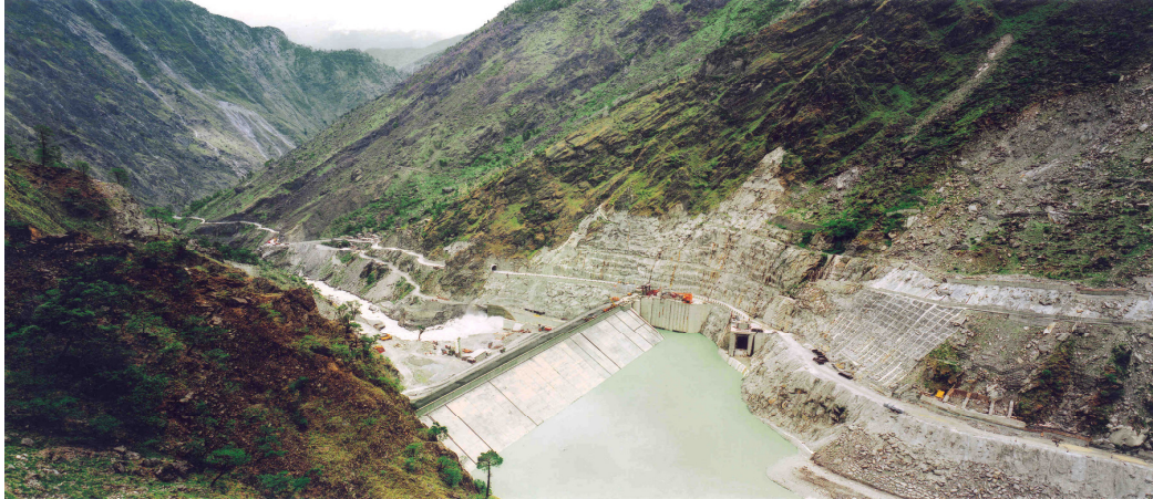
Dam view upstream of 280 MW Dhauliganga Project
