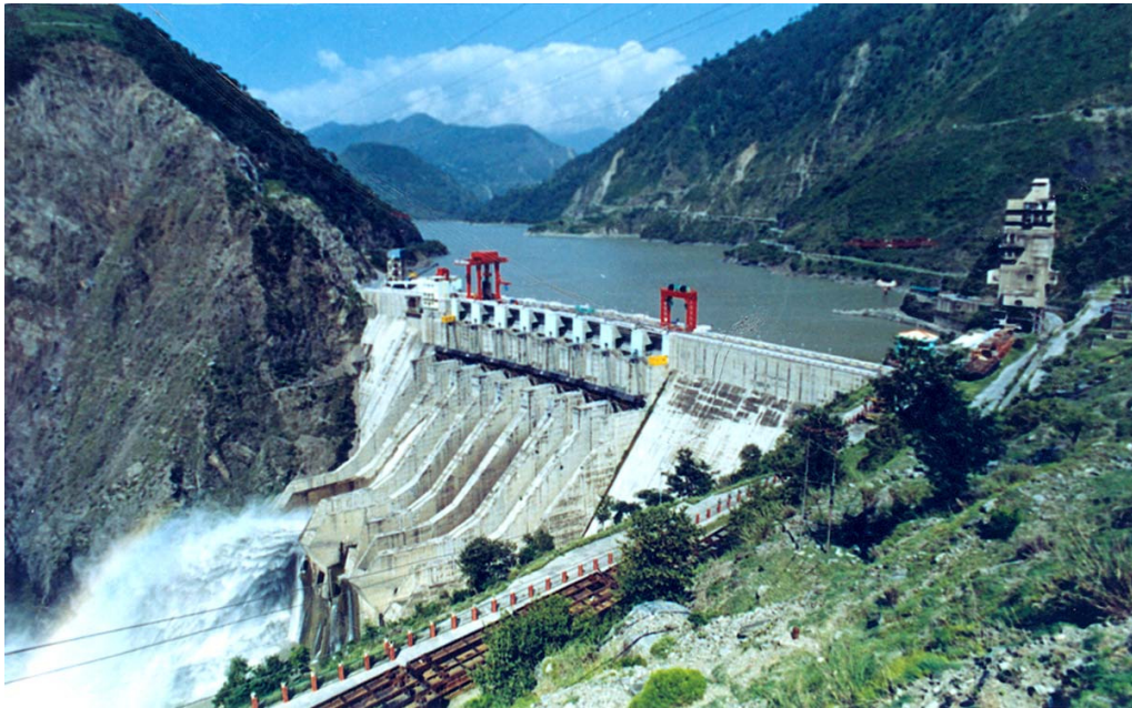
Dam View of 540 MW Chamara Stage-I H. E. Project
