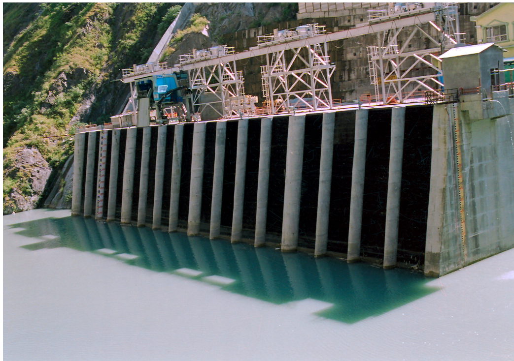
Intake Structure of 1500 MW Nathpa Jhakri H. E. Project
