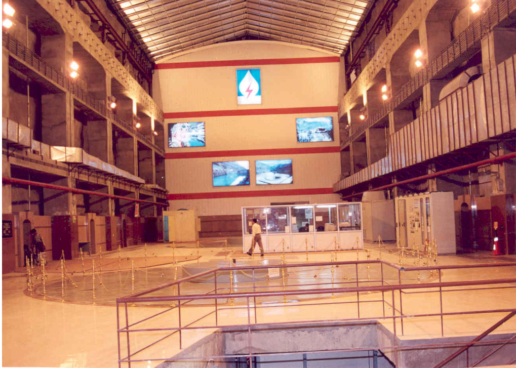
Machine Hall of 1500 MW Nathpa Jhakri Project
