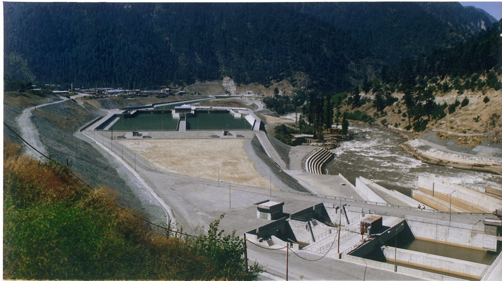
Panoramic view of 1000 MW Indira Sagar Project
