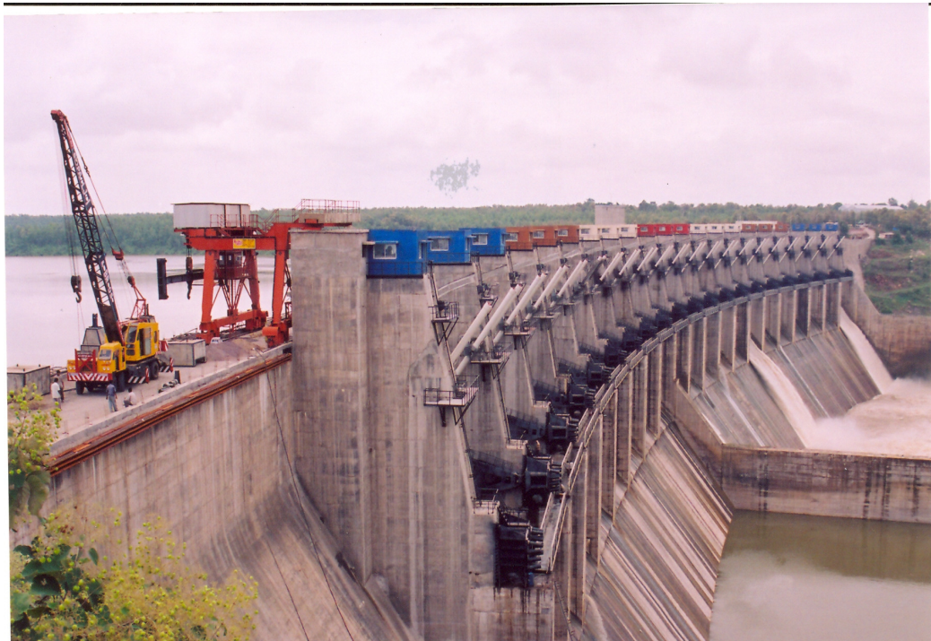
Dam Side View of 1000 MW Indira Sagar Project
