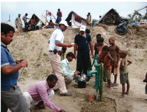
Handpump installation in a disaster affected area.
