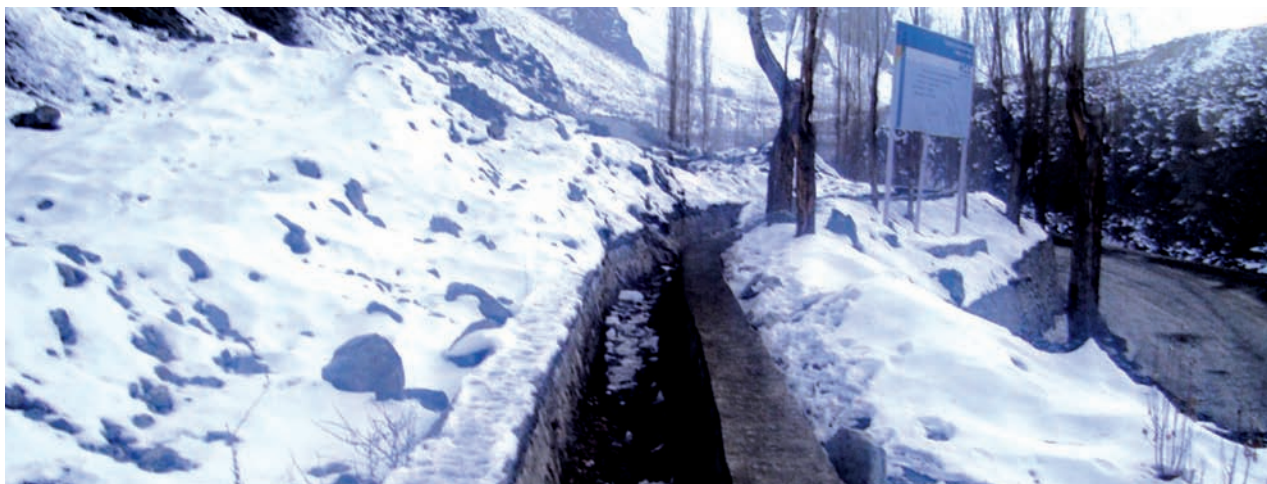
Kul Restoration at Chutak Hydro Power Project, Jammu & Kashmir.
