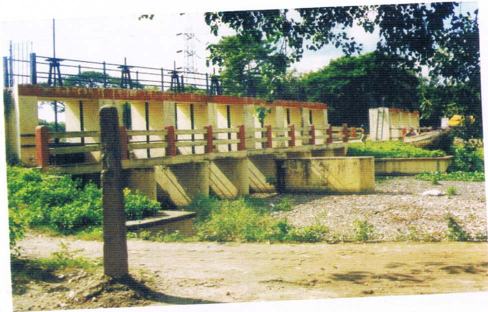
Lock gate at the confluence of Calcutta outfall canals on river Kulti
