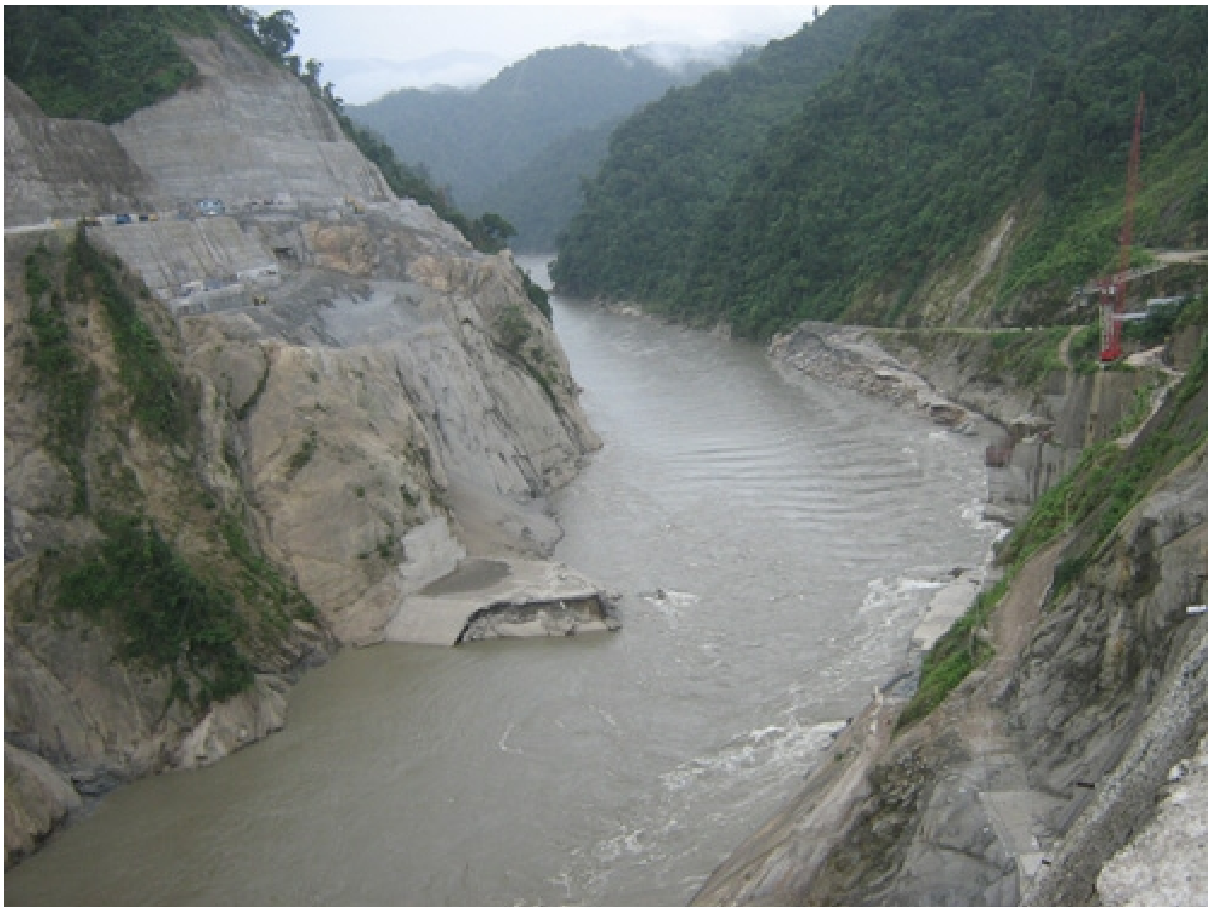
Collapse of the coffer dam of the Lower Subansiri HEP on June 13, 2008(Courtesy : PMSBV)
