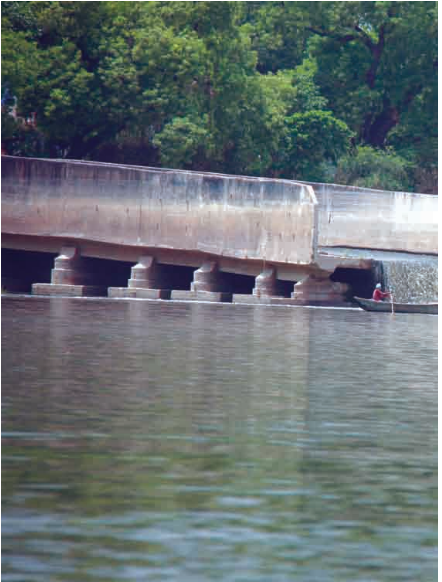
Government estimates show that almost 3 billion litres of sewage (partially treated and untreated) is discharged into Ganga everyday from cities, thereby severely degrading the water quality
