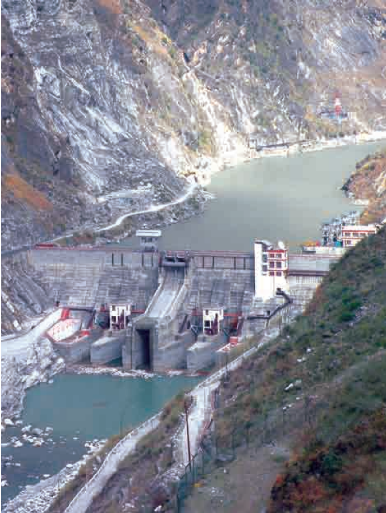
Run-of-the-river hydropower projects leads to diminishing flows in the river length for which the water has been diverted through tunnels
