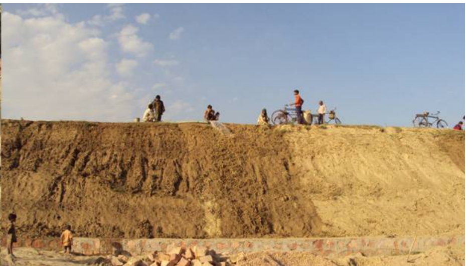
Preparation of slopes for inclined wall
