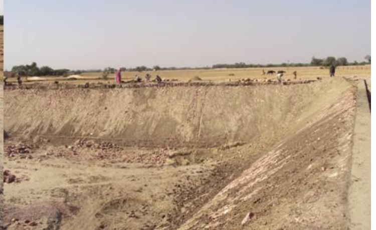
Construction of upper supporting wall
