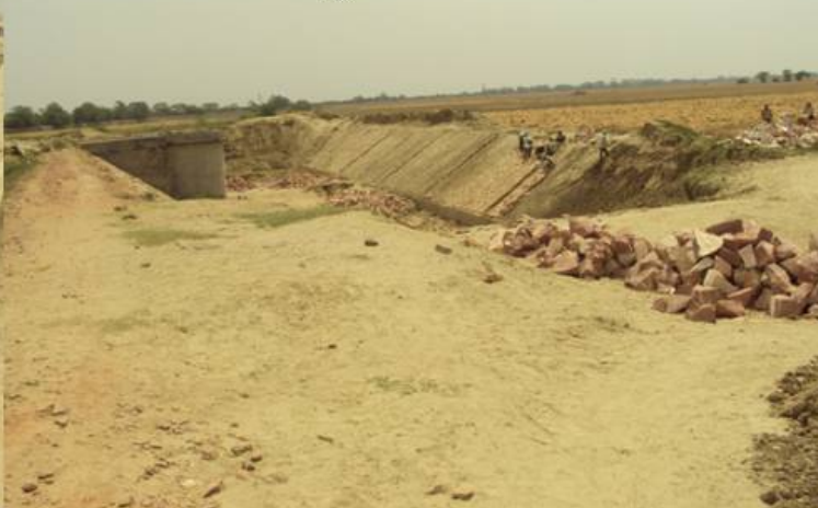
Pitching inclined wall
