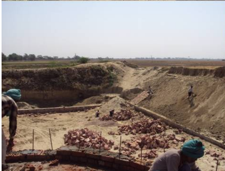
Pitching inclined wall
