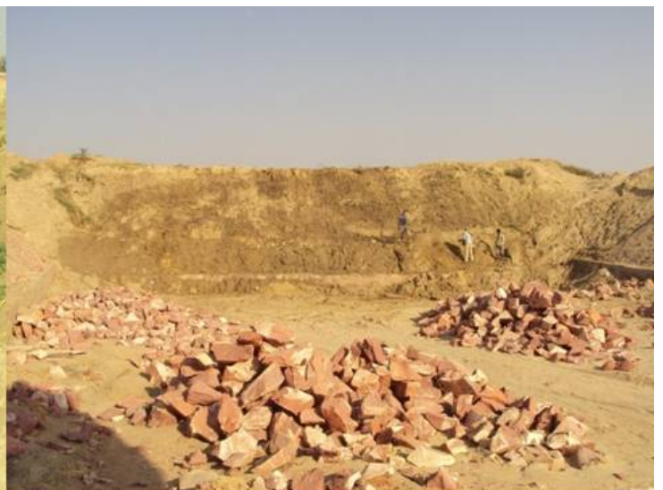
Preparation of slopes for inclined wall
