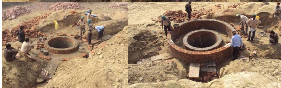
Foundation of supporting wall
