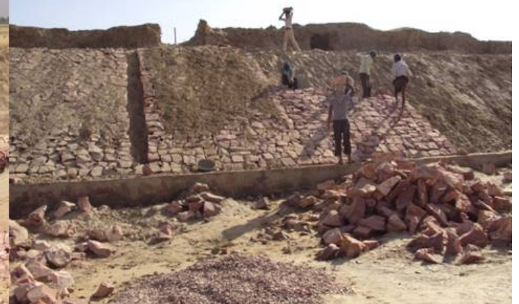
Pitching inclined wall
