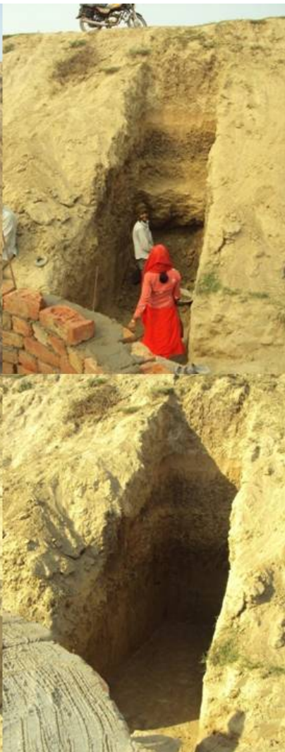
Base for the Bridge
