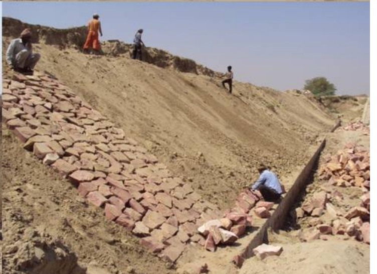
Pitching inclined wall
