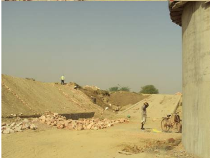
Pitching inclined wall
