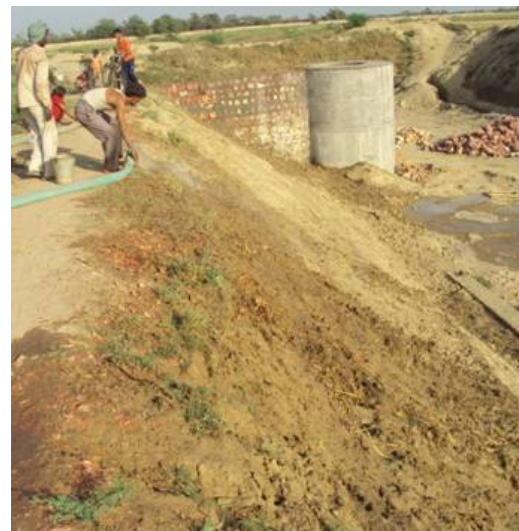
Preparation of slopes for inclined wall
