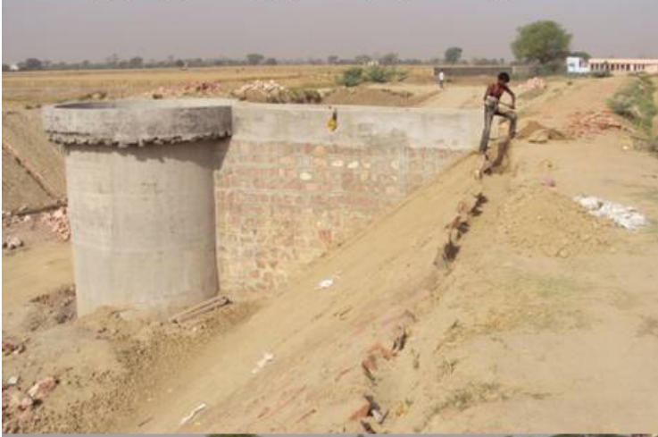
Digging for upper supporting wall
