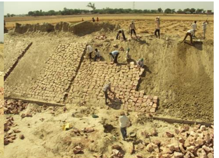
Pitching inclined wall
