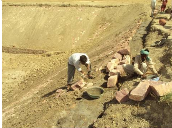
Construction of upper supporting wall
