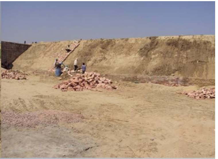
Pitched inclined wall
