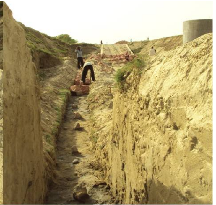
Foundation of supporting wall (Opp. to well side)
