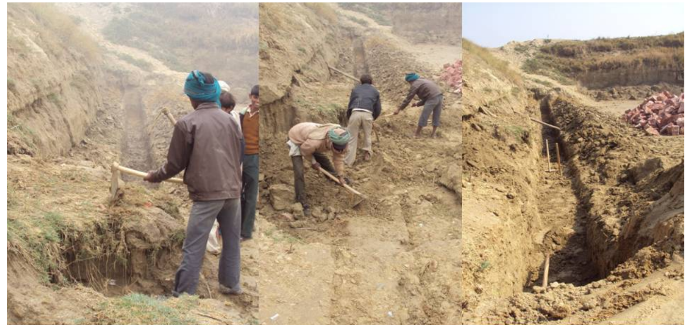
Digging for the foundation of supporting wall
