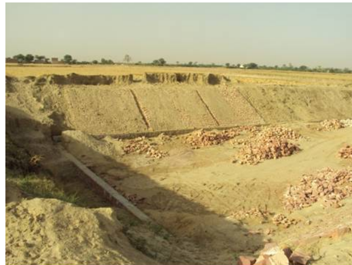
Pitching inclined wall
