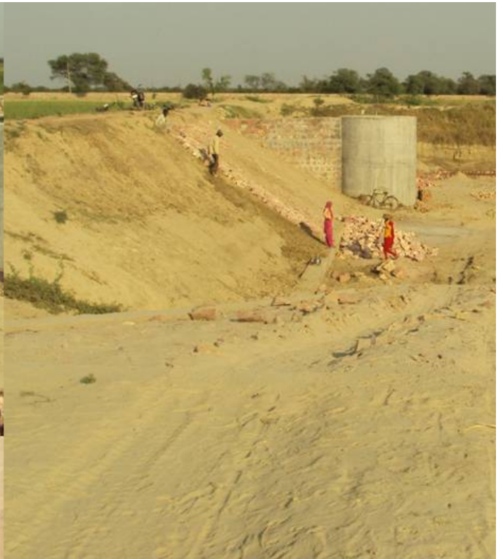
Pitching inclined wall
