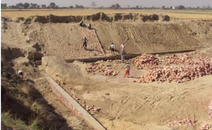
Pitching inclined wall
