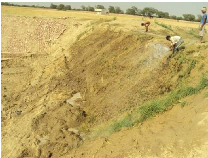
Preparation of slopes for inclined wall
