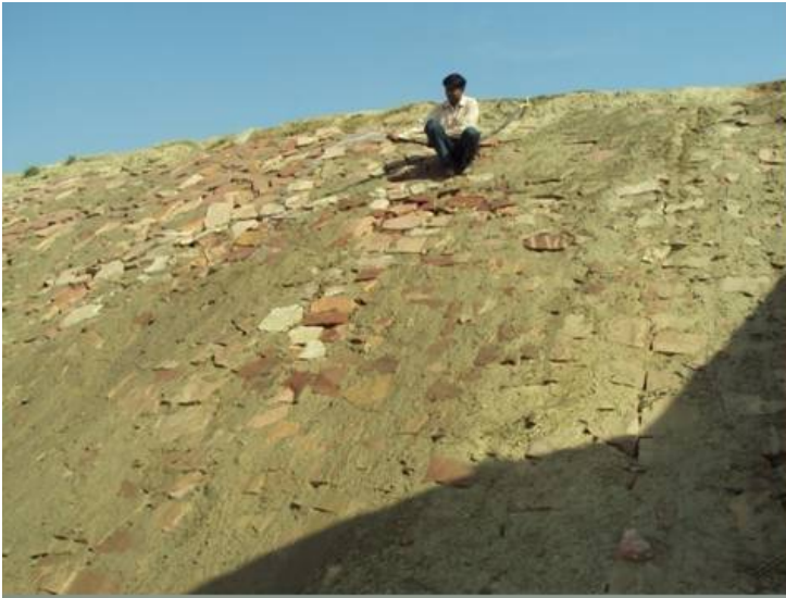
Pitched inclined wall
