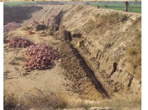
Digging for the foundation of supporting wall
