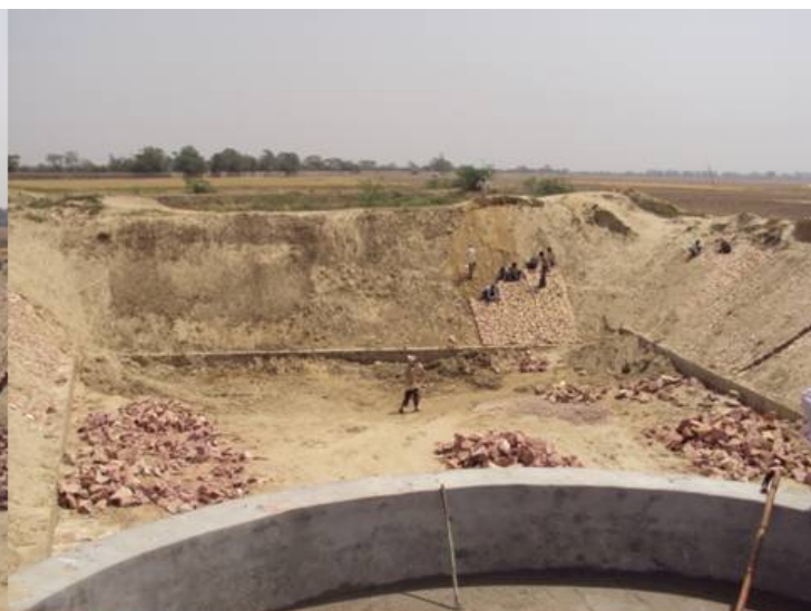
Pitching inclined wall
