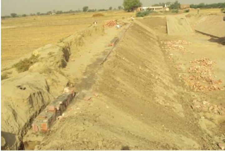
Construction of upper supporting wall
