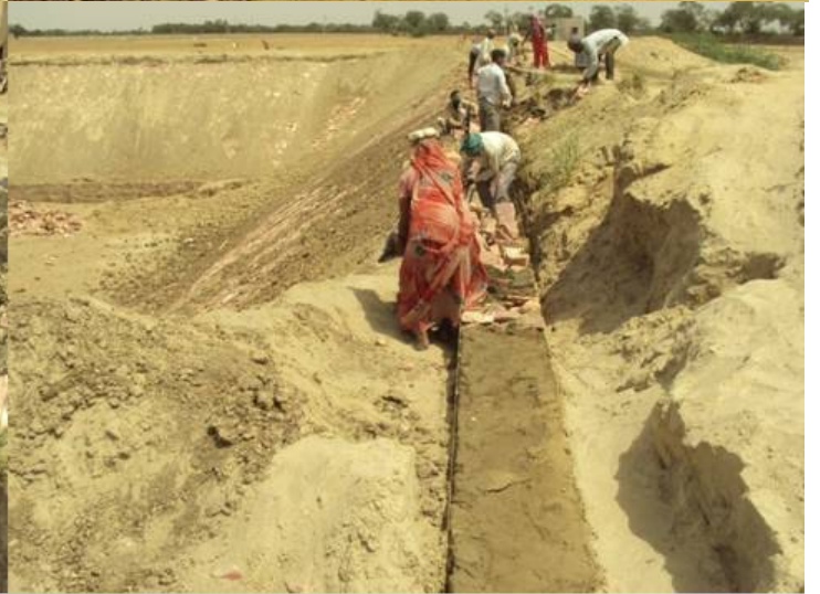
Construction of upper supporting wall
