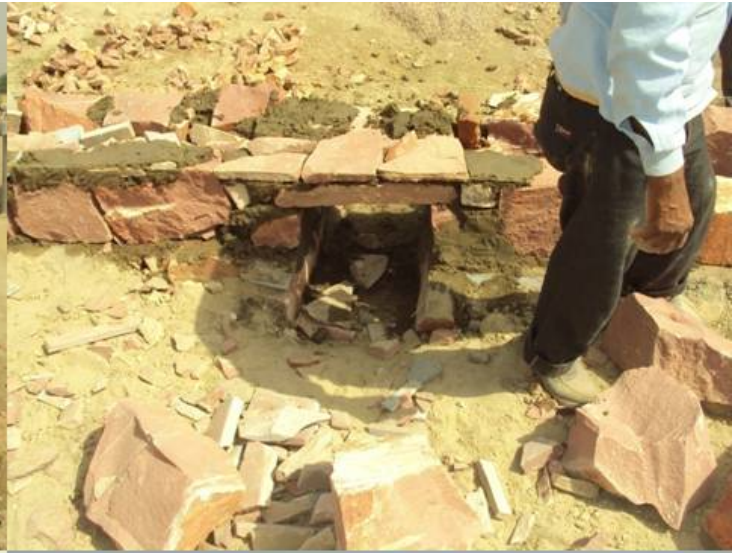
Construction of upper supporting wall
