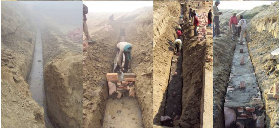
Foundation of supporting wall
