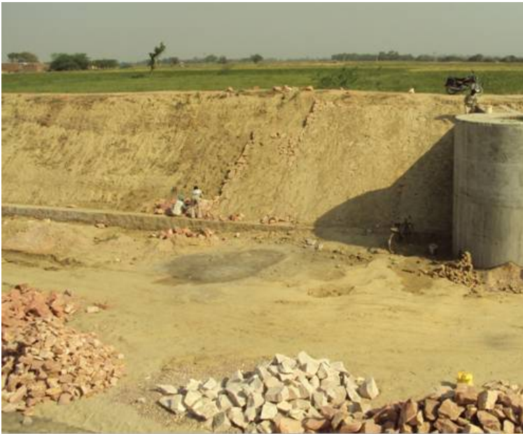
Pitching inclined wall
