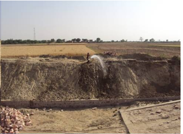
Pitching inclined wall
