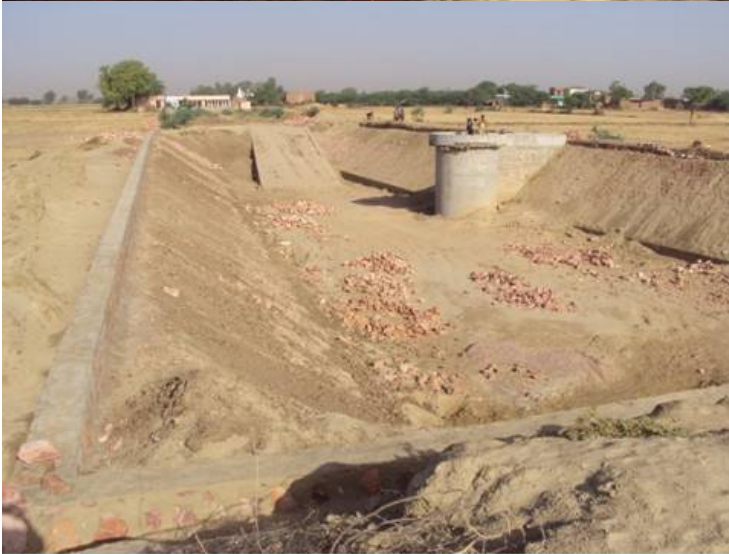
Construction of upper supporting wall
