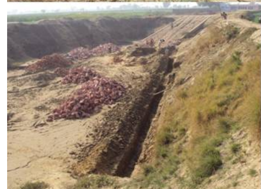
Digging for the foundation of supporting wall
