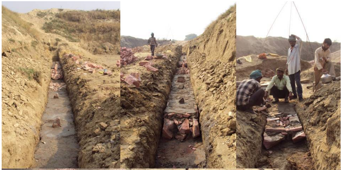
Foundation of supporting wall
