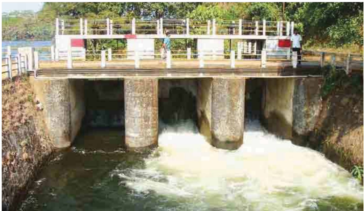
Barrage on Valappattanam River, Kerala. © Rajeev Raghavan
