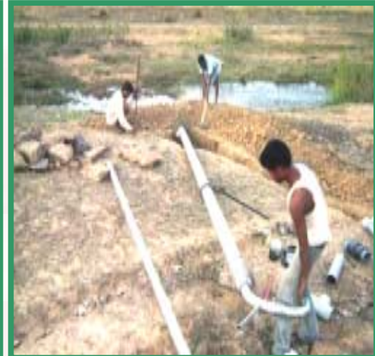
Laying underground pipe
