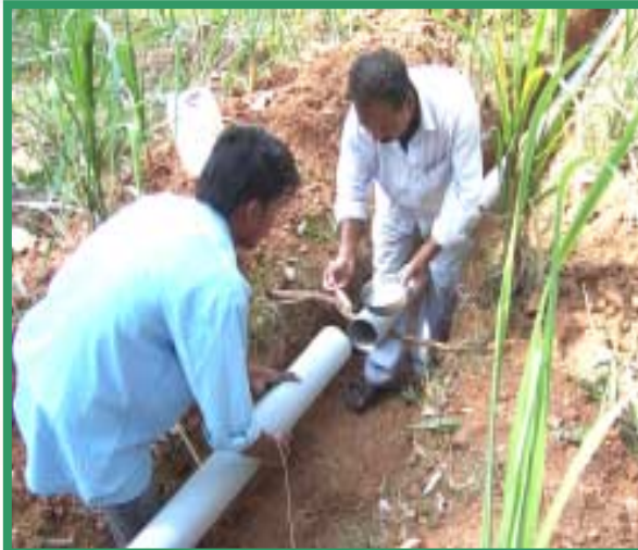
Laying underground pipe
