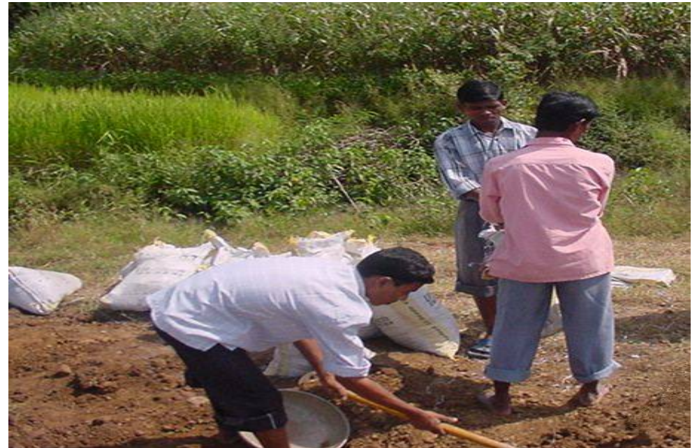
Construction of Vanrai bandhara with the help of community
