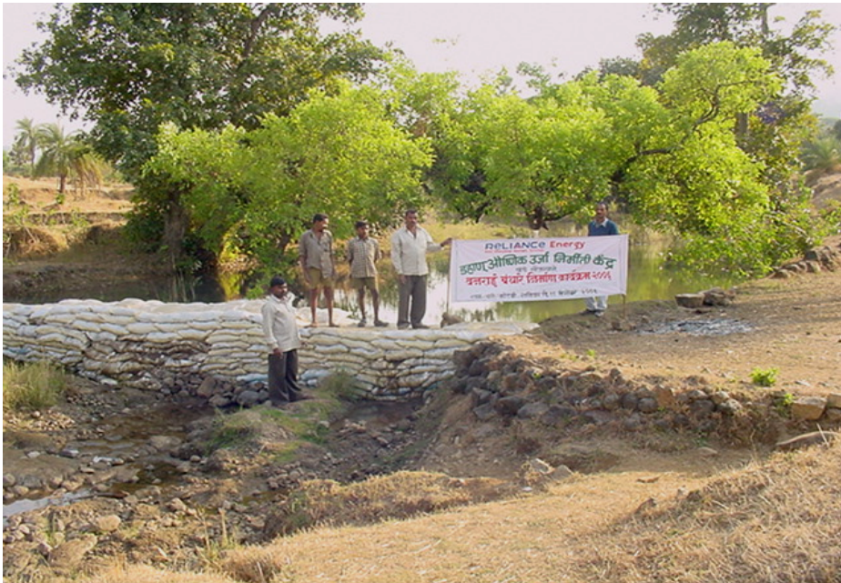
Construction of Vanrai bandhara with the help of community
