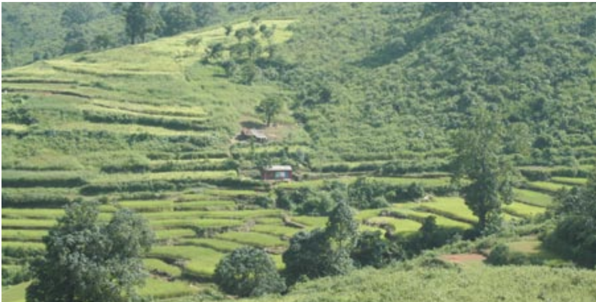
Nestling in the hills: the power house of Putsil
