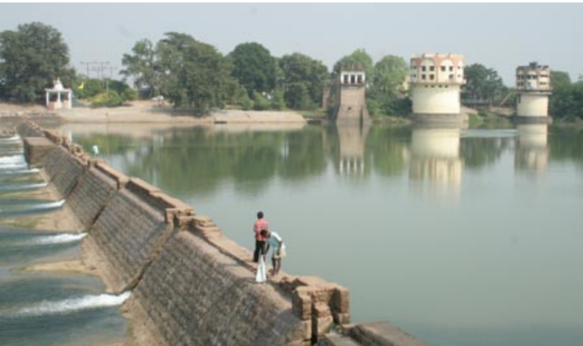
Anicut and pump houses at Sheonath rive
