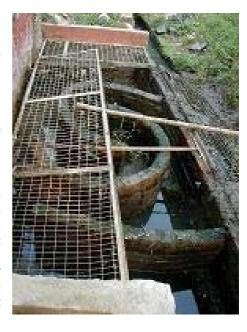
kernel fibres and wood coal with stone and boulders as filters. The overall cost of the plant came to around Rs.7.0 Lakhs, plant capacity at 35Kl per day.
