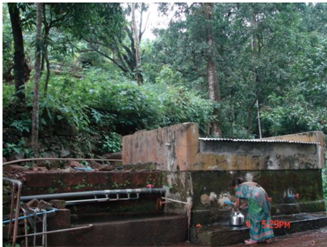
Spring tank with individual water connections
