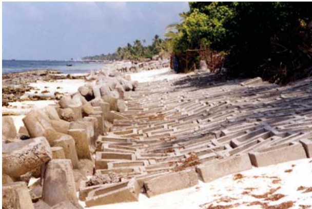
Figure 9.12: Concrete revetments to control the wave run up disturb the natural beach profile at Kadamat Island reef area located in the Arabian Sea
