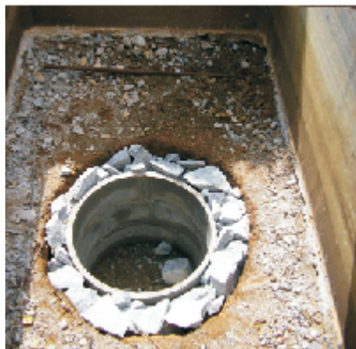
Recharge well inside the sump
