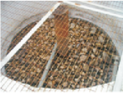
Recharge well around bore-well
