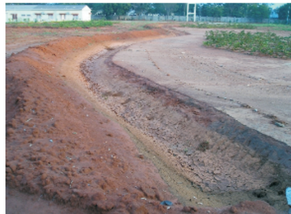
Swale directing the rainwater falling on the land to a recharge well
