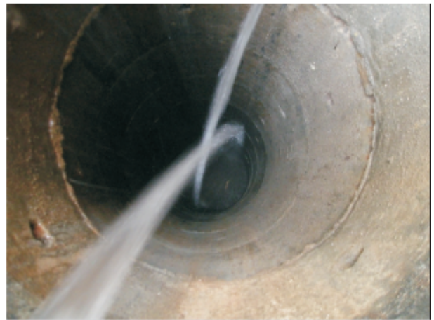
Rainwater being sent for recharge
