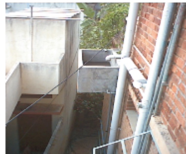
Ferro cement tank
