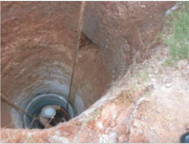
RCC rings being placed
