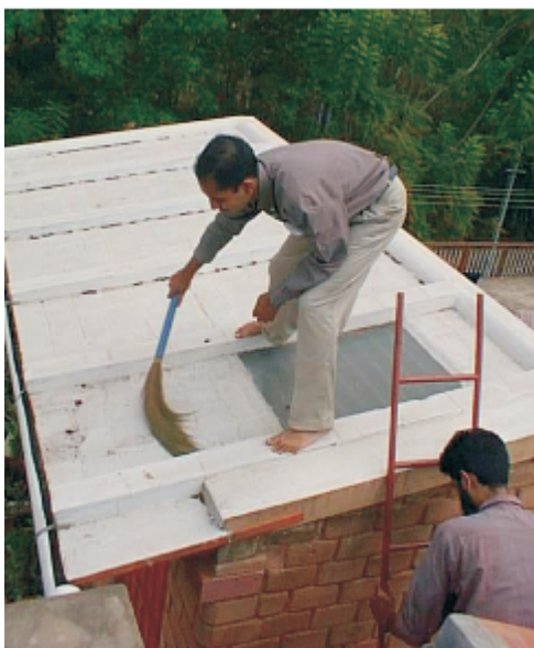
Maintenance of the roof is simple and crucial
