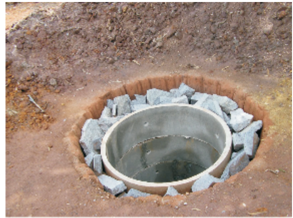
Recharge well with filtering material around (jelly)
