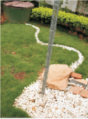
Chains leading the water to a recharge well
