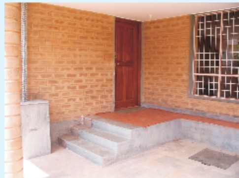
Filter and sump tank integrated at the entrance
