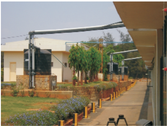
Rain barrels collecting rooftop rainwater
