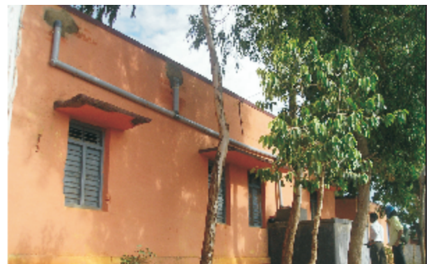
Sloping roof & Flat Roof
