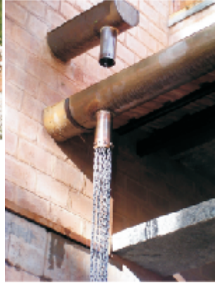
Gutter/chains connection details
