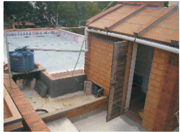
Rooftop Rainwater harvesting
