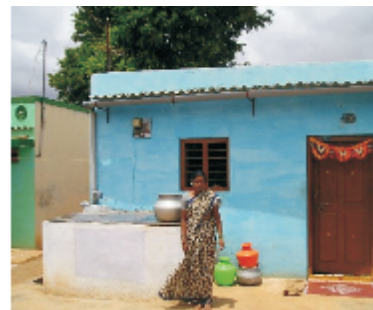
Above ground masonry tank
