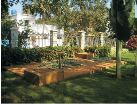
Sump tank converted into rainwater storage tank
