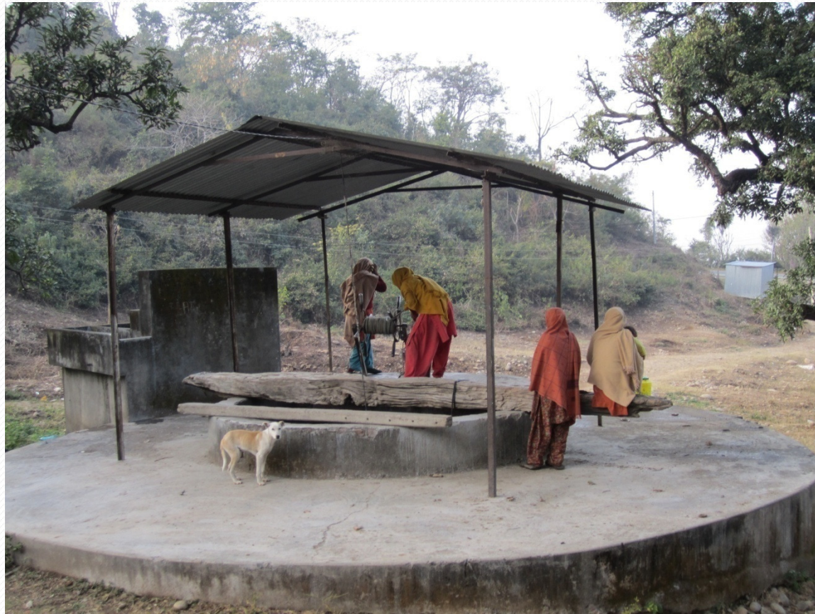
Renovation of Well
