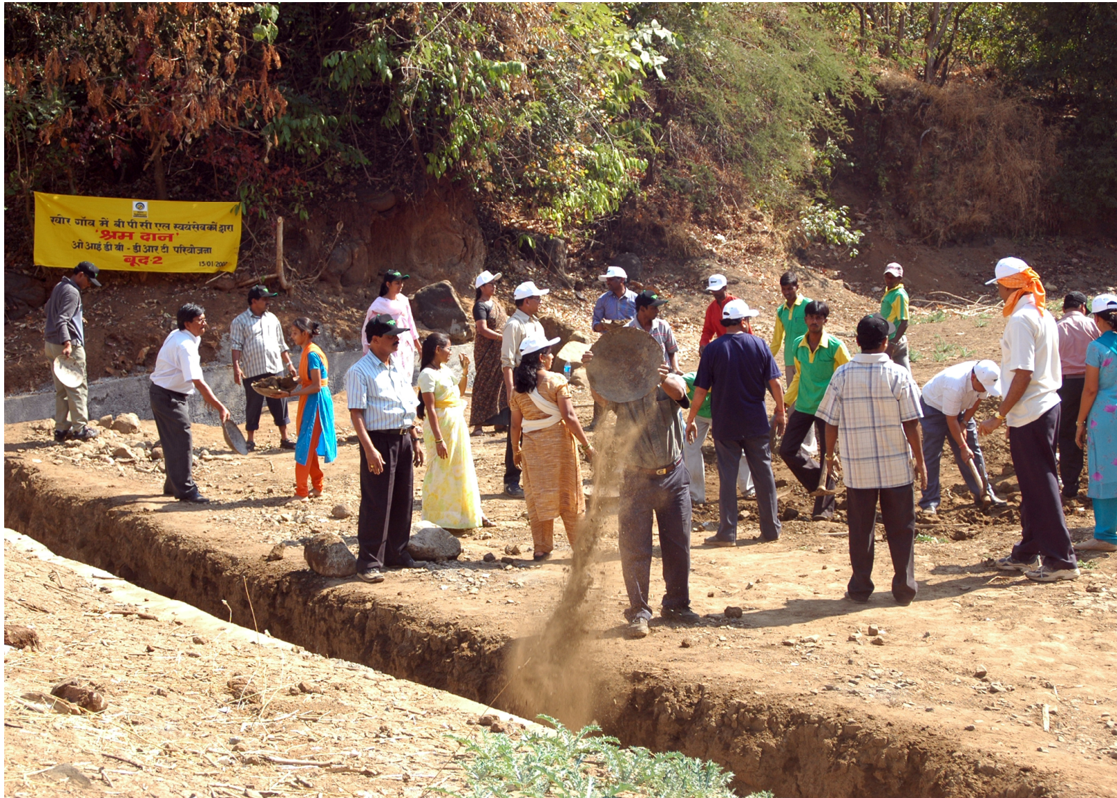
BOOND II --- BPCL employees volunteering in village Khor
