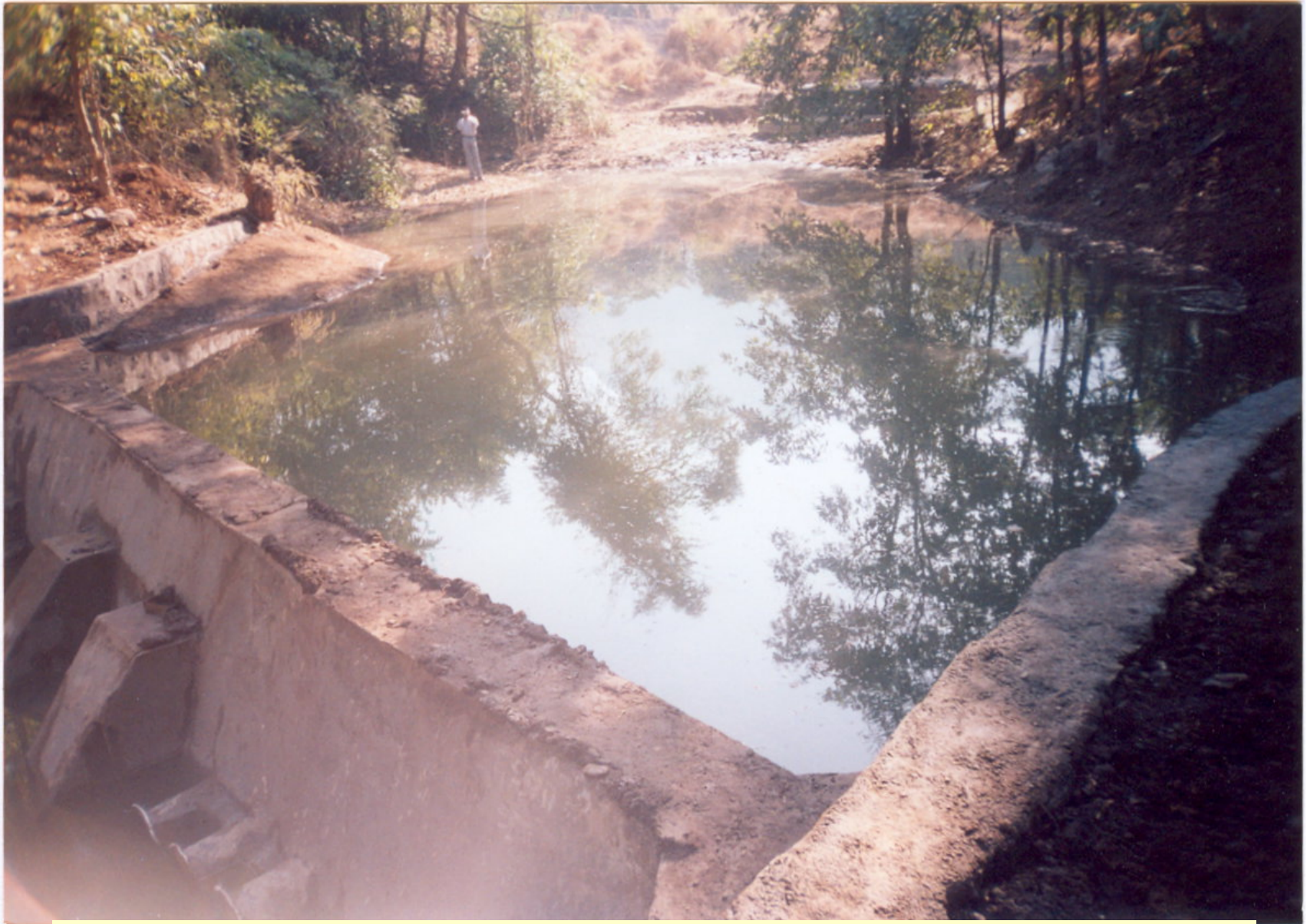
BOOND II --- Supporting Bund in village Khor
