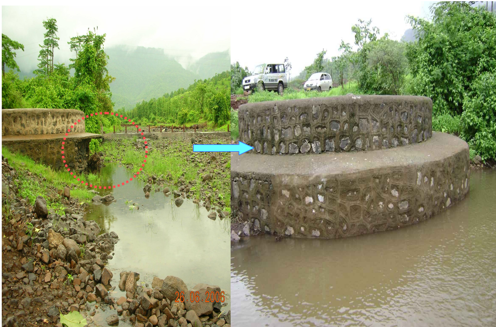
BOOND II --- Well Revival in Mahuli
