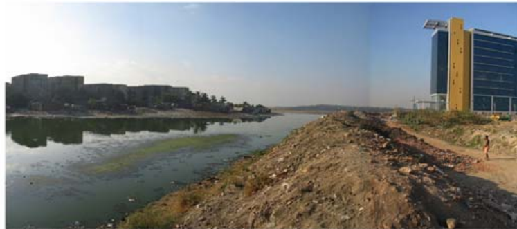
Before transformation: Debris dumping along the edges of Quibble Island, creek polluted with wastewater & garbage
