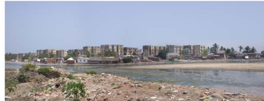
Before transformation: Debris dumping along the edges of Quibble Island, overlooking encroachments in Srinivasapuram with edges covered by garbage
