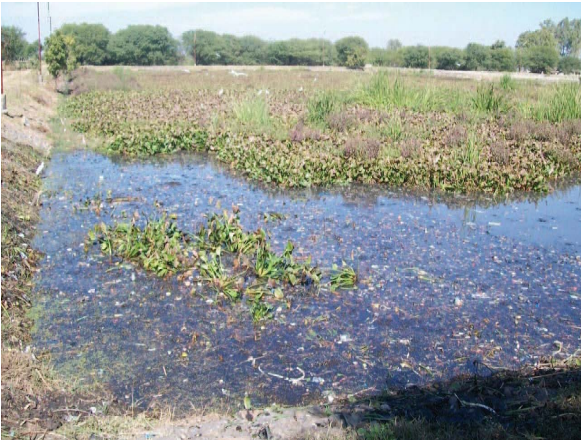
Sewage accumulation due to waste stabilisation pond not being cleaned in for STP, Kshipra River, Ujjain
