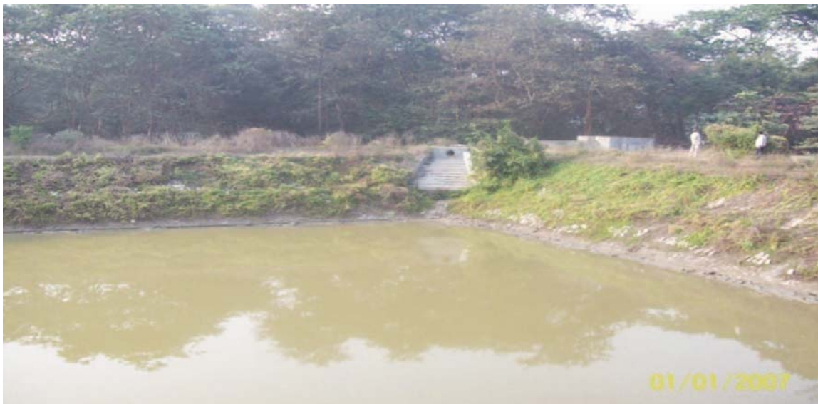
Non functional STP at Halilshar
