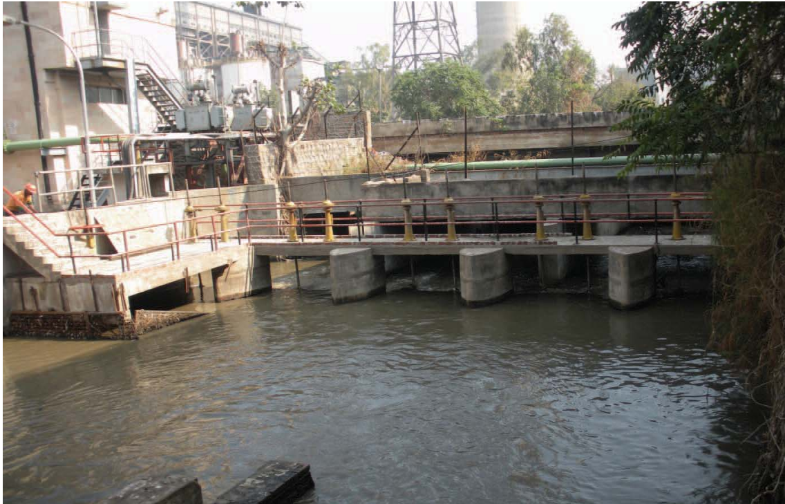
10 mld STP at Delhi Gate nallah (Untreated sewage passing into yamuna)
