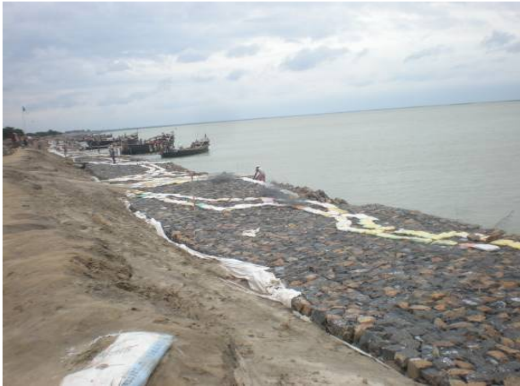
A view of execution of anti-erosion work at downstream of Manikchakghat 2011
