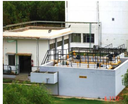
SEWAGE TREATMENT PLANT
