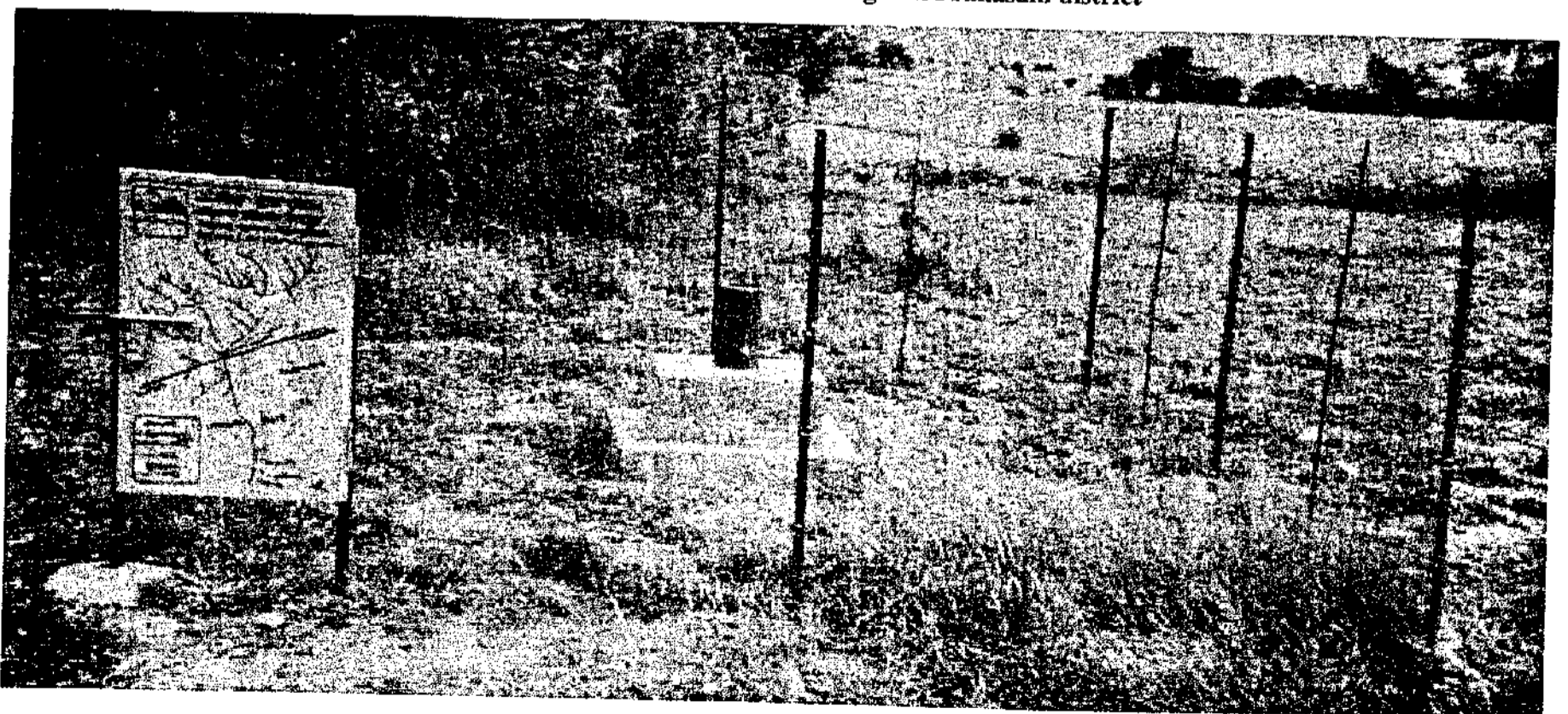
Figure 3-10: A rain gauge station at one of the PHM villages in Prakasam district
