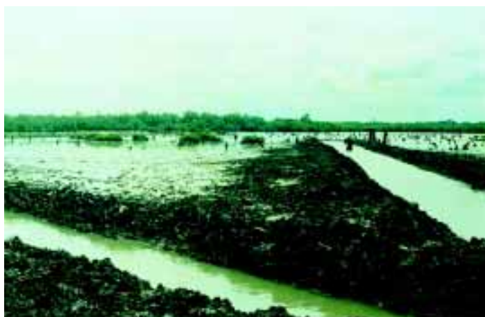
Figure 2.14 A view of the canals constructed in the degraded area (1994)
