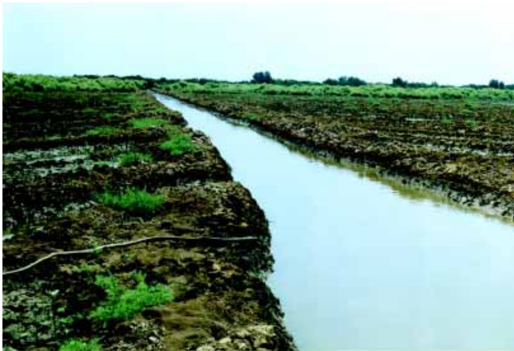
Figure 2.17 Canals constructed in the restoration site for free tidal flushing
