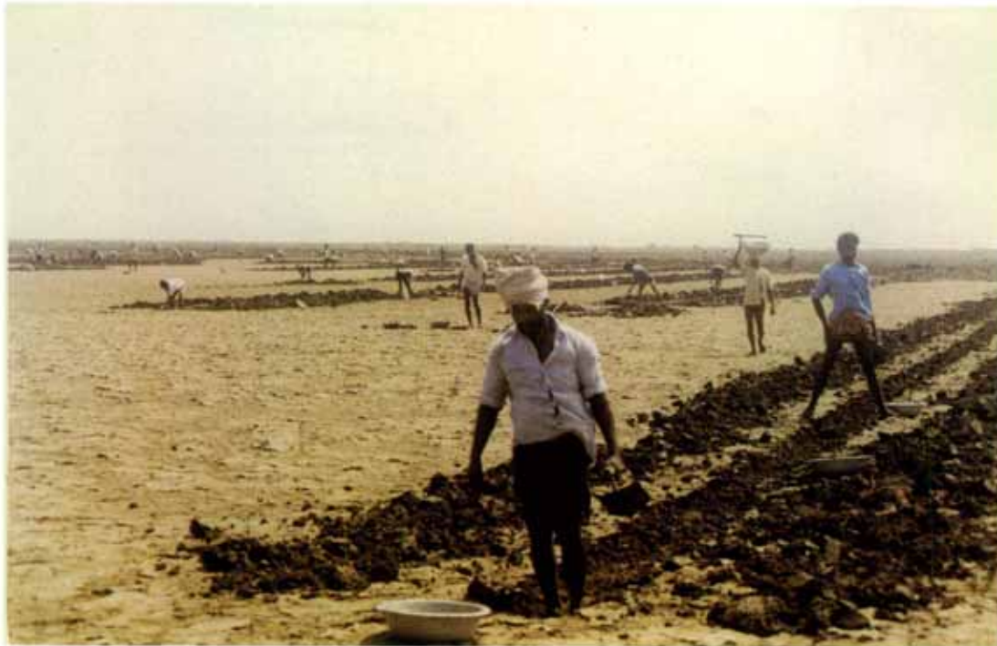
Figure 55. Canal construction in degraded mangroves
