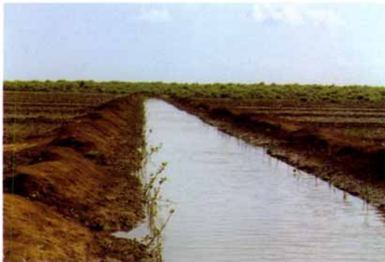
Figure 56. Nursery (top) and canal construction (bottom) in Sorlagondi RF
