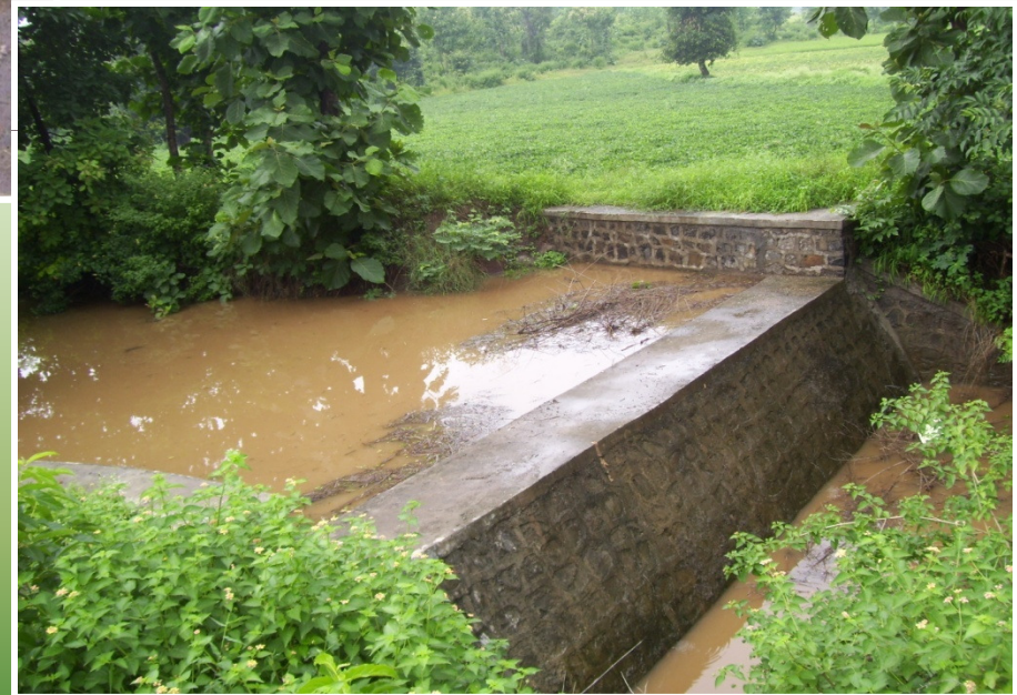
Cement Nala Bund
