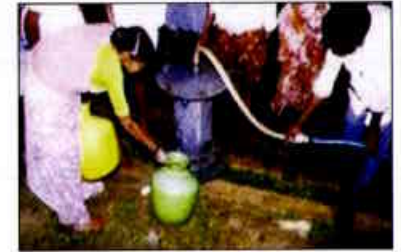
Figure 6.1: Nitrate Removal Systems of Ion Exchange India Limited
