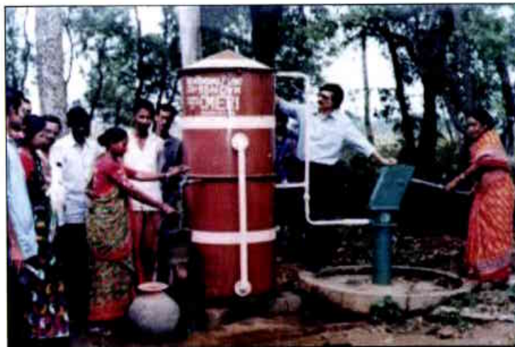
Figure 5.2: CMERI iron removal plant
