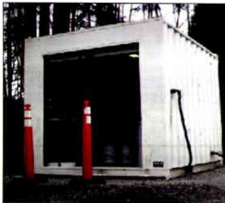
Figure 5.13: "IRON STOPPER" Containerized Treatment System, including the "DEFERUM™" hydroautomatic filter
