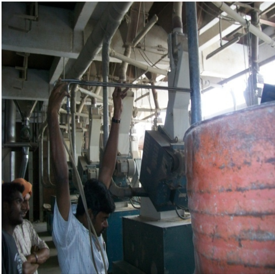
Fig.6.9. Outlet from Single Huller (Port Hole 4) on 3 rd floor
