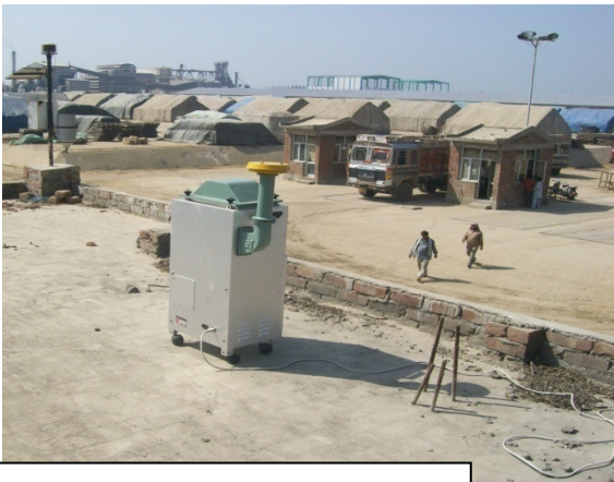
Fig.6.13 Near Factory Gate
