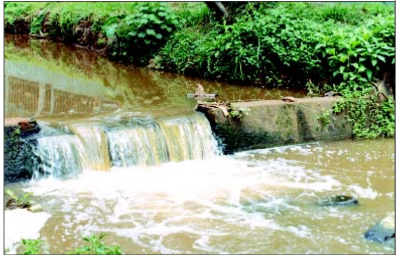
Plate 16. A weir constructed across an urban river to promote oxygen transfer to the water for enhanced degradation of pollutants.
