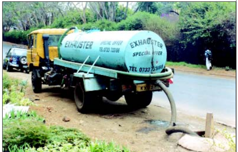
Plate 20. A cesspit evacuation tanker or exhauster vehicle emptying raw sewage in a main sewer line through an open manhole. Exhauster services are in high demand in areas without sewerage network.
