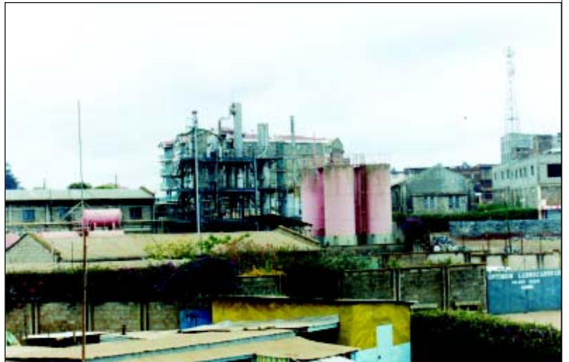
Plate 24. A recycling plant for used engine oil located in Kikuyu town west of Nairobi. The oil is collected from motor vehicle service stations in the city and transported to the facility for processing.
