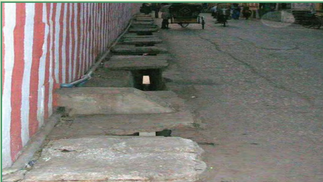
Work relating to covering of storm water drains, Tirupati
