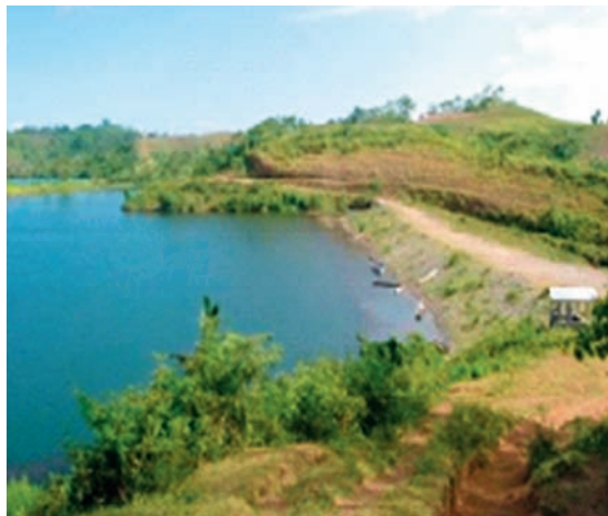
Figure 6.4. Small Water Impounding System in the Philippines
