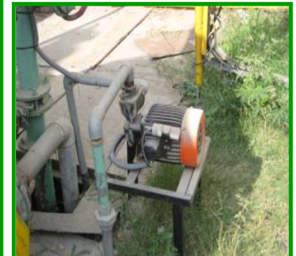
Closed water loop for Cooling
