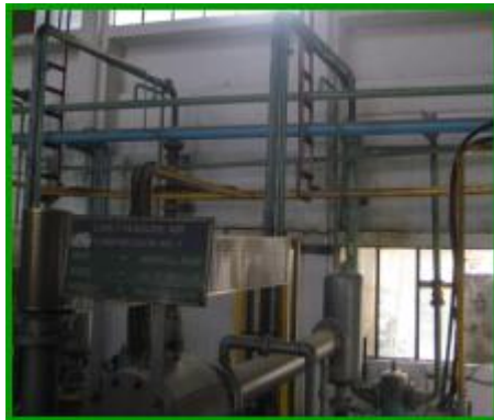
Closed Water Loop system, Interconnection of water pipe lines, DG Set & Air Compressor Cooling System
