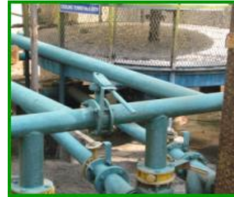
Closed Water Loop system, Interconnection of water pipe lines, DG Set & Air Compressor Cooling System
