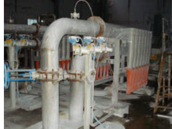
Picture after modification Water requirement : 4m 3 /hr
