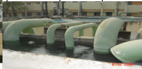
Treated Water Recycled as CW make-up
