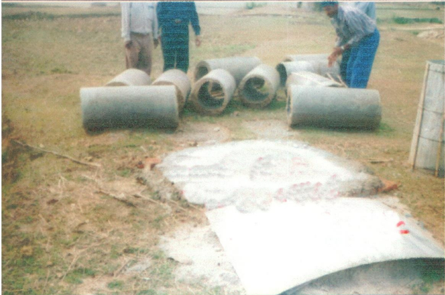
Hume Pipe constructed by SHG
