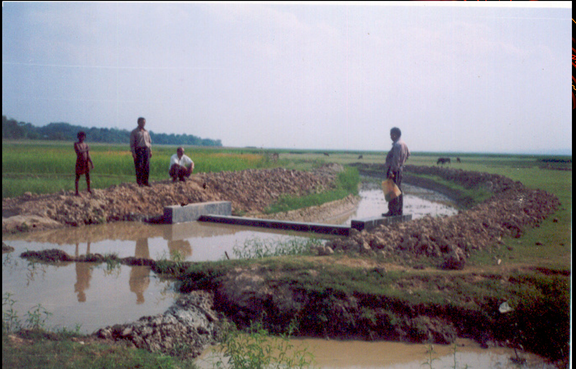
Reexcavation of Drainage Channel at Jyostnakuri visited by D.O.S.C. (PIA) which benefitted 40 Ha. Of Agri Land
