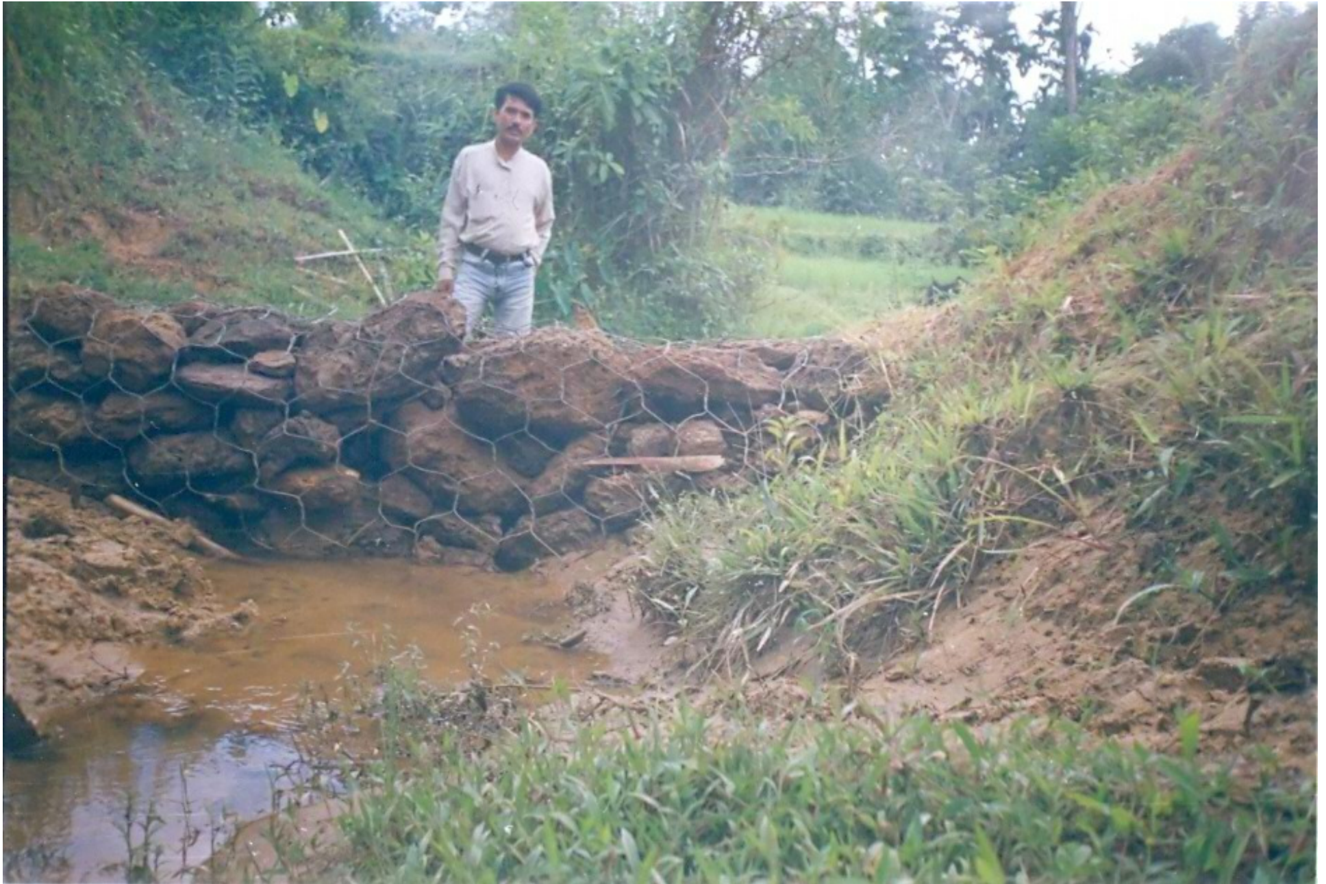
Drainage line Treatment with wire crates
