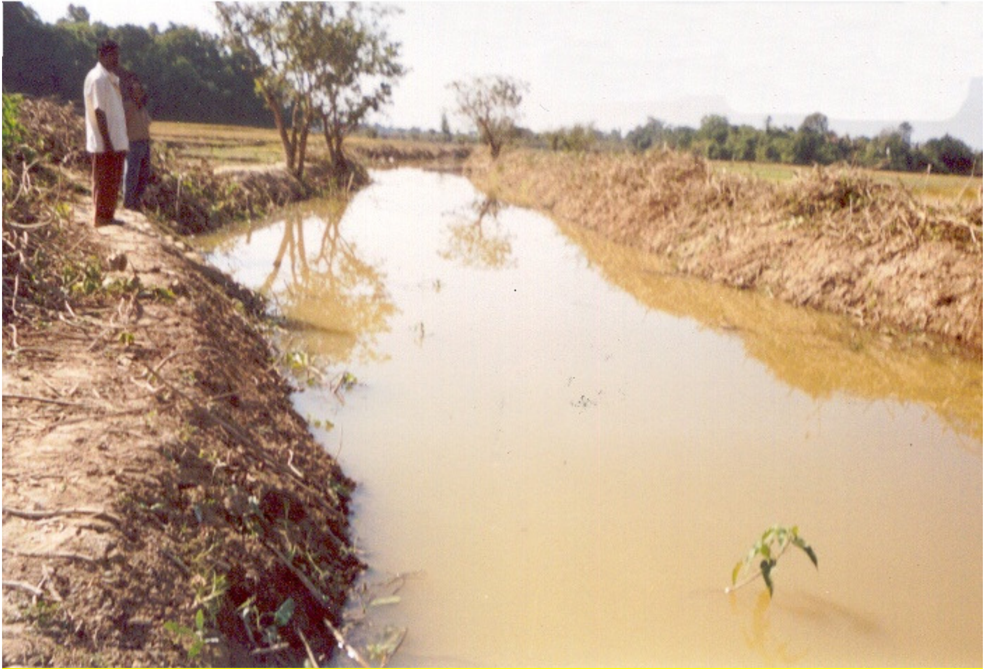
Excavation of Drainage Channel at Chinanalcherra, benefitted 9 Ha.of Land
