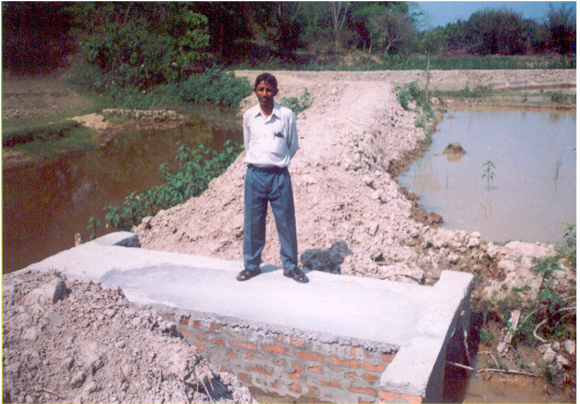
Contour Graded Bund with Culvert at Chinanalcherra, area benefited 25.0 Ha.
