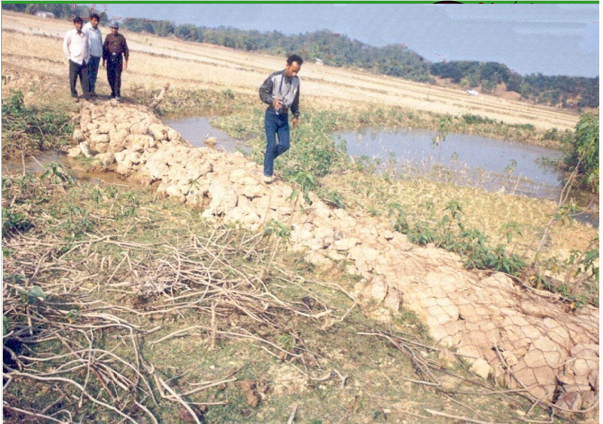
Boulder Check-Dam at Bakalkandi benefitted 12 Ha. Of Agri Land.
