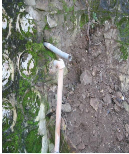
View of Cracked Pushta and Broken Intake Pipeline at Dhaur Barsudi WSS
