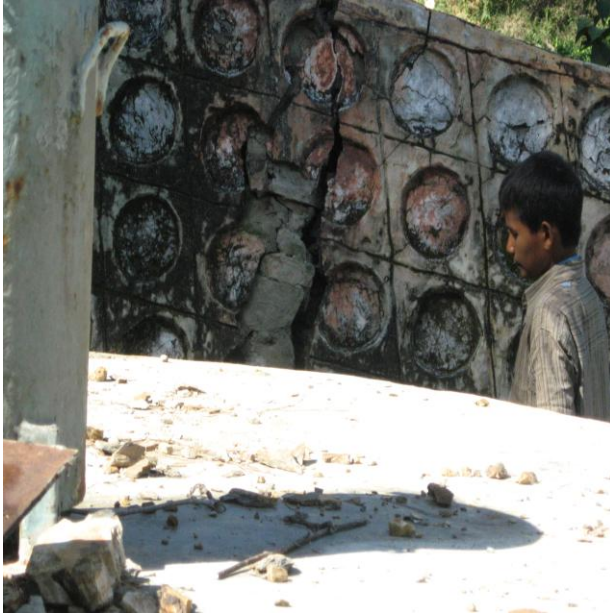
View of Cracked Pushta and Broken Intake Pipeline at Dhaur Barsudi WSS
