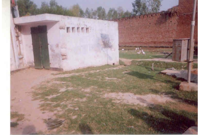
Incomplete construction of OHT and Pumphouse at VWSC Godhi, Moradabad District
