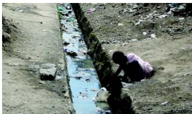
Fig. 1. A child collects drinking water from a cracked municipal supply pipe directly above an open sewer in the Nakuru slum district of Kenya. In order to collect the treated water from the pipe, her container is partially immersed in raw sewage.
