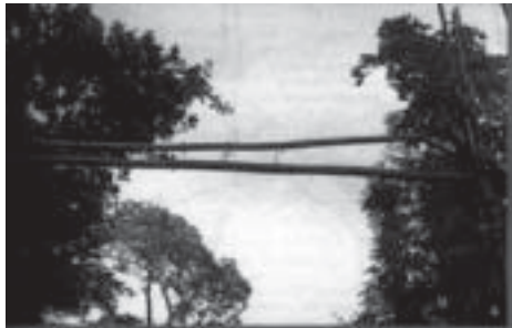
Pix 4 : if the pipes pass a road, they are taken high above the land.
