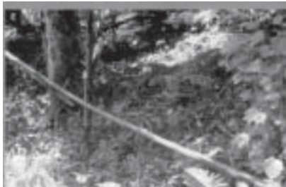
Pix 4 : if the pipes pass a road, they are taken high above the land.
