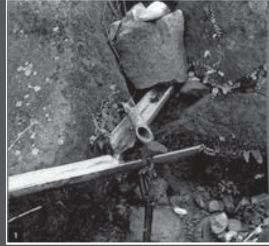
Pix 1: Bamboo pipes are used to divert perennial springs on the hilltops to the lower reaches by gravity
