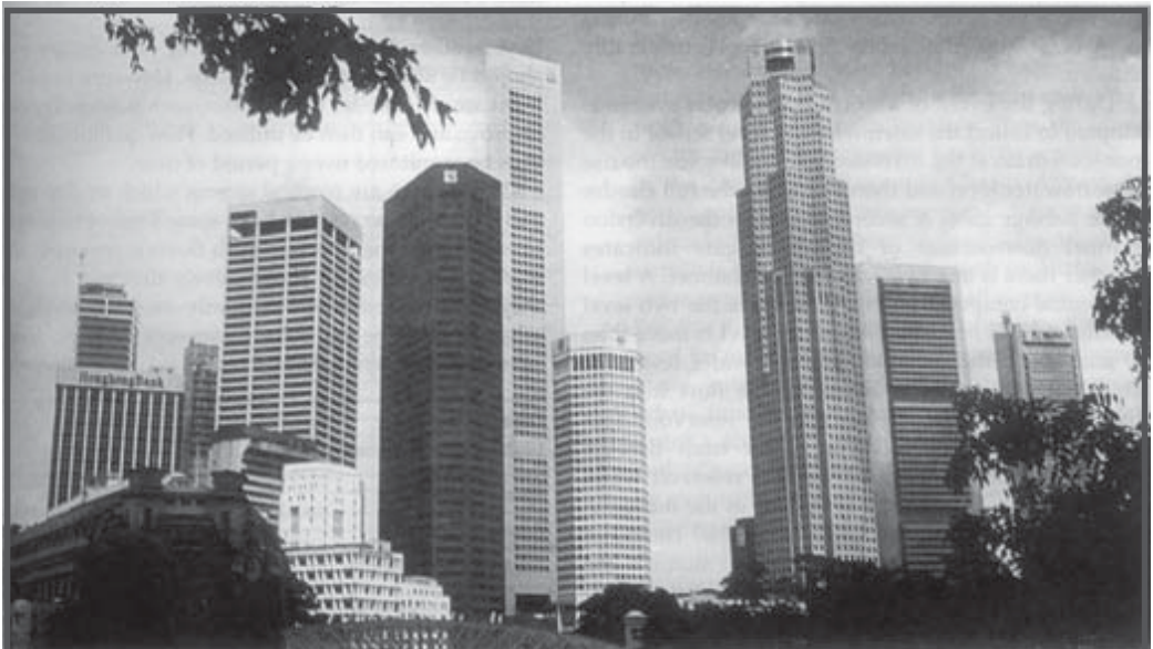
Skyscrapers catching water from the sky in Singapore. Almost 50 Per cent of the land serves as a catchment area
