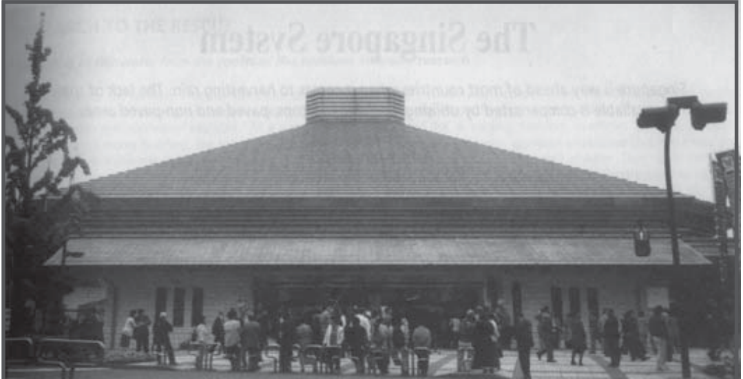
Rainwater harvesting is gathering momentum in Japan as a solution to deal with flooding and water shortage. At Ryogoku Kokugikan, Tokyo's famous Sumo wrestling arena, 70 percent of the facilities, including the air conditioning system and toilets, Use rainwater collected from its roof
