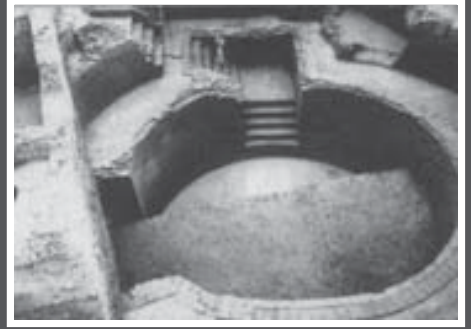
TANK C: The third tank was circular, with an elaborate staircase allowing access to low water levels, its spill and exit channels led away from this. Its bed had a series of wells in case the tank dried up.
