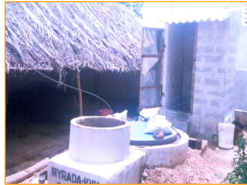
Bio Gas unit
