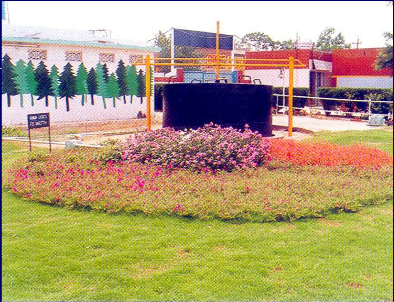
Public toilets linked with biogas plant (with gas holder)
