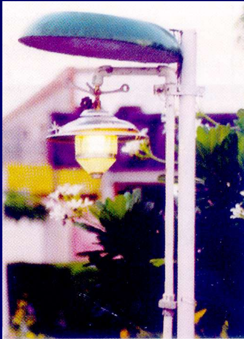
Use of biogas for mantle lamps
